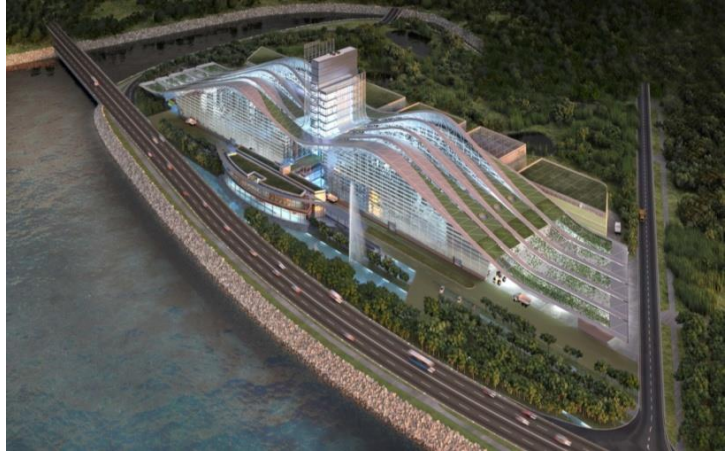
Sludge Treatment Facility Hong Kong
